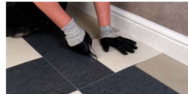
Figure 5 Measuring using an overlapping tile
